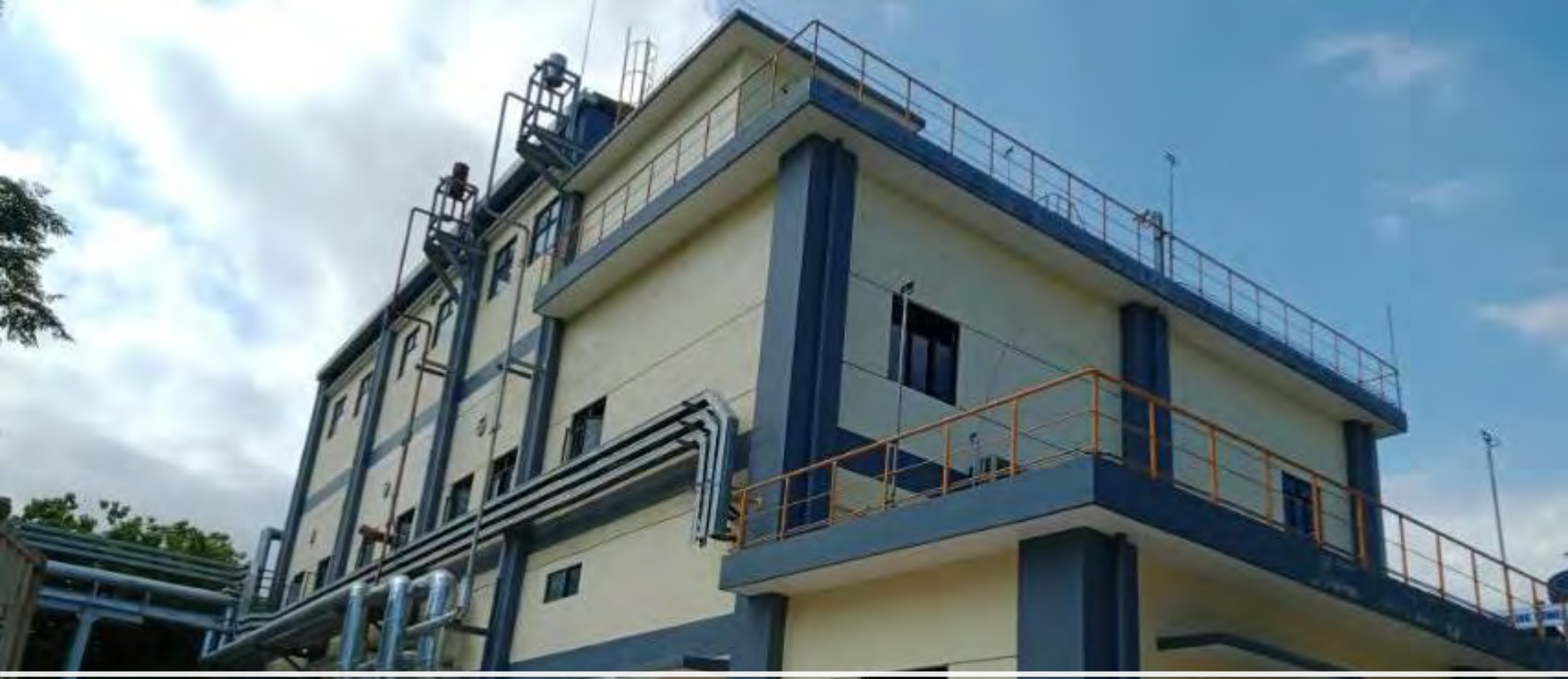
Heat Recovery facility in APO Cement Plant
