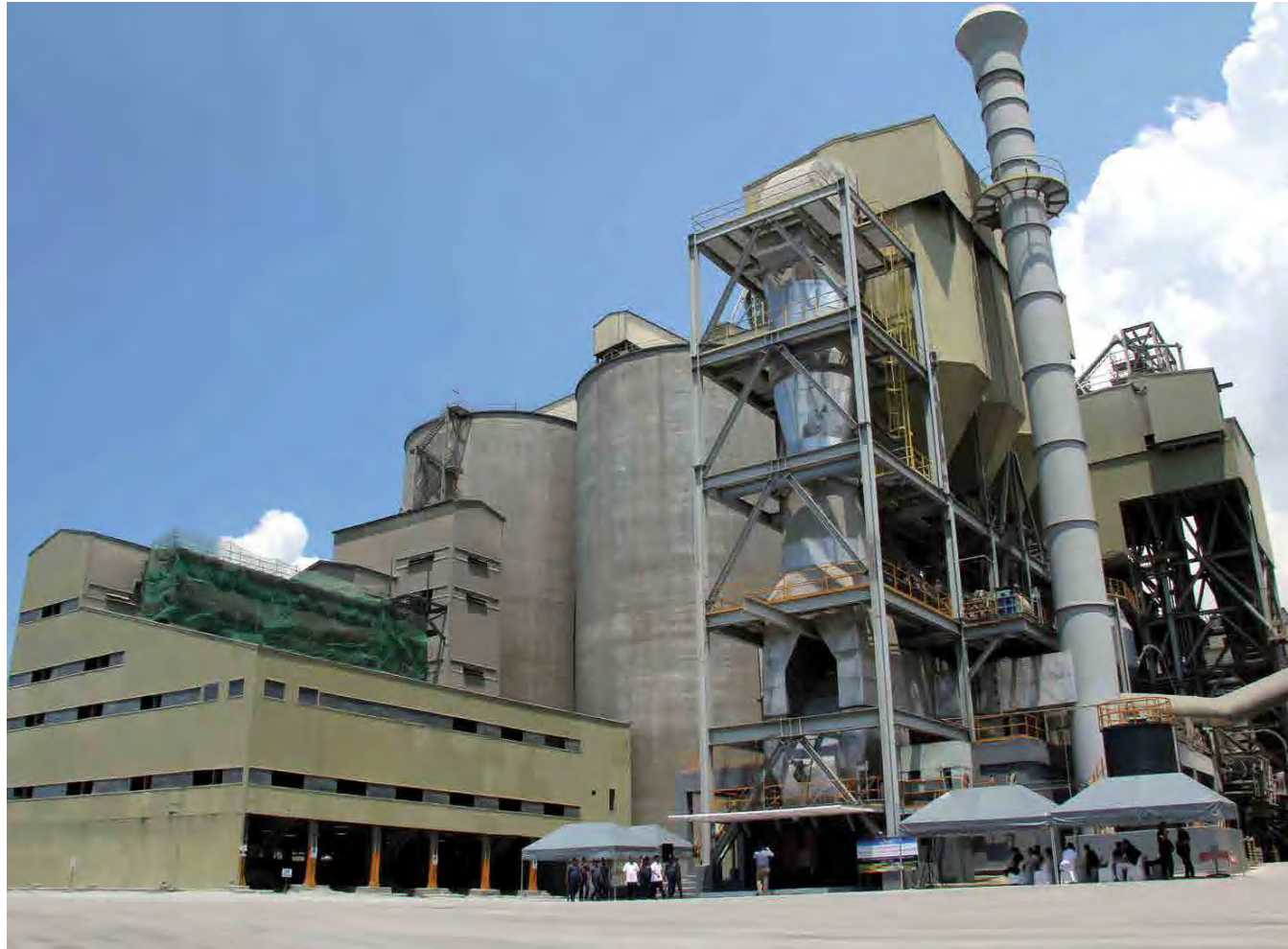
Vertical Cement Mill in APO Cement Plant
