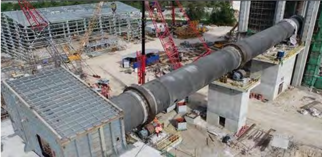
New rotary kiln at Solid Cement Plant
