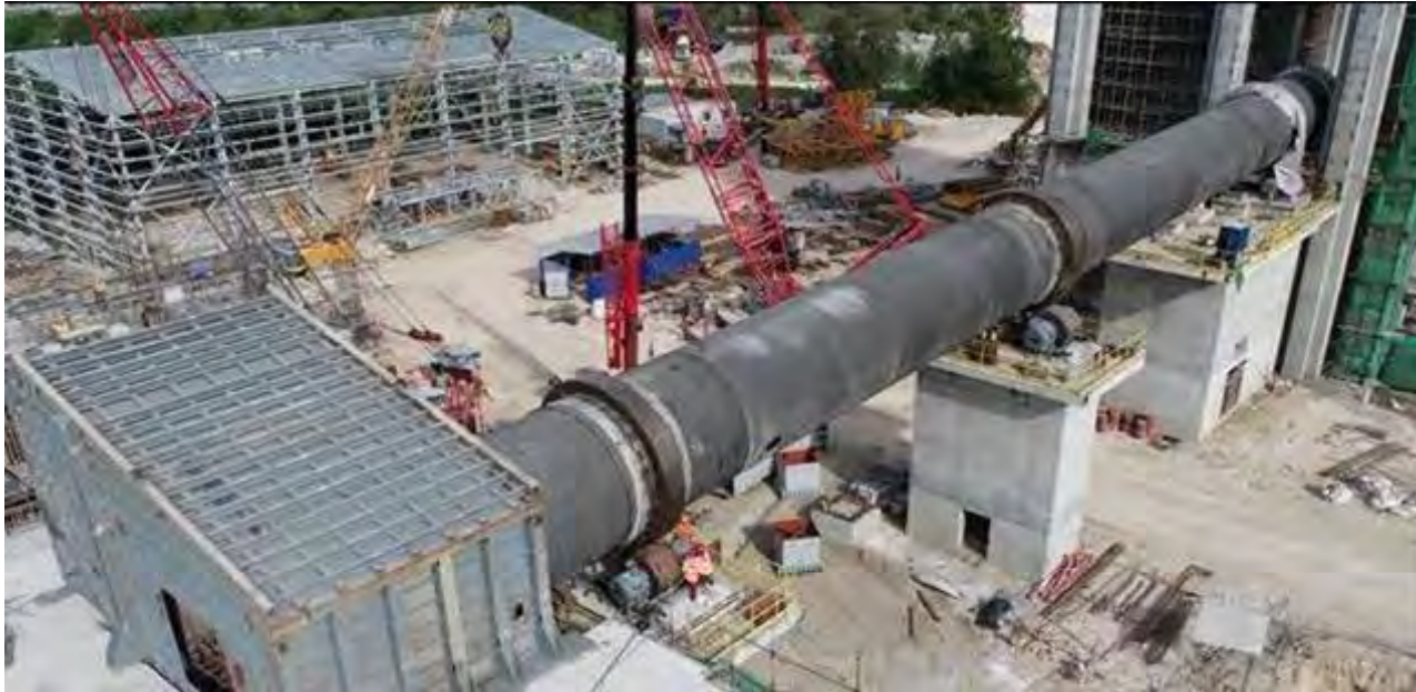
Lifting of new rotary kiln into position at Solid Cement Plant (Jan. 2021)
