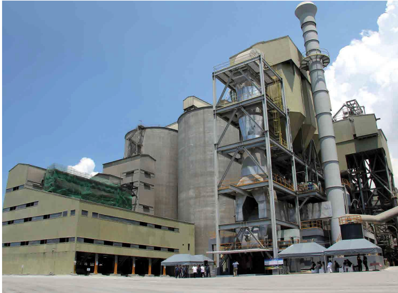
Vertical Cement Mill in APO Cement Plant
