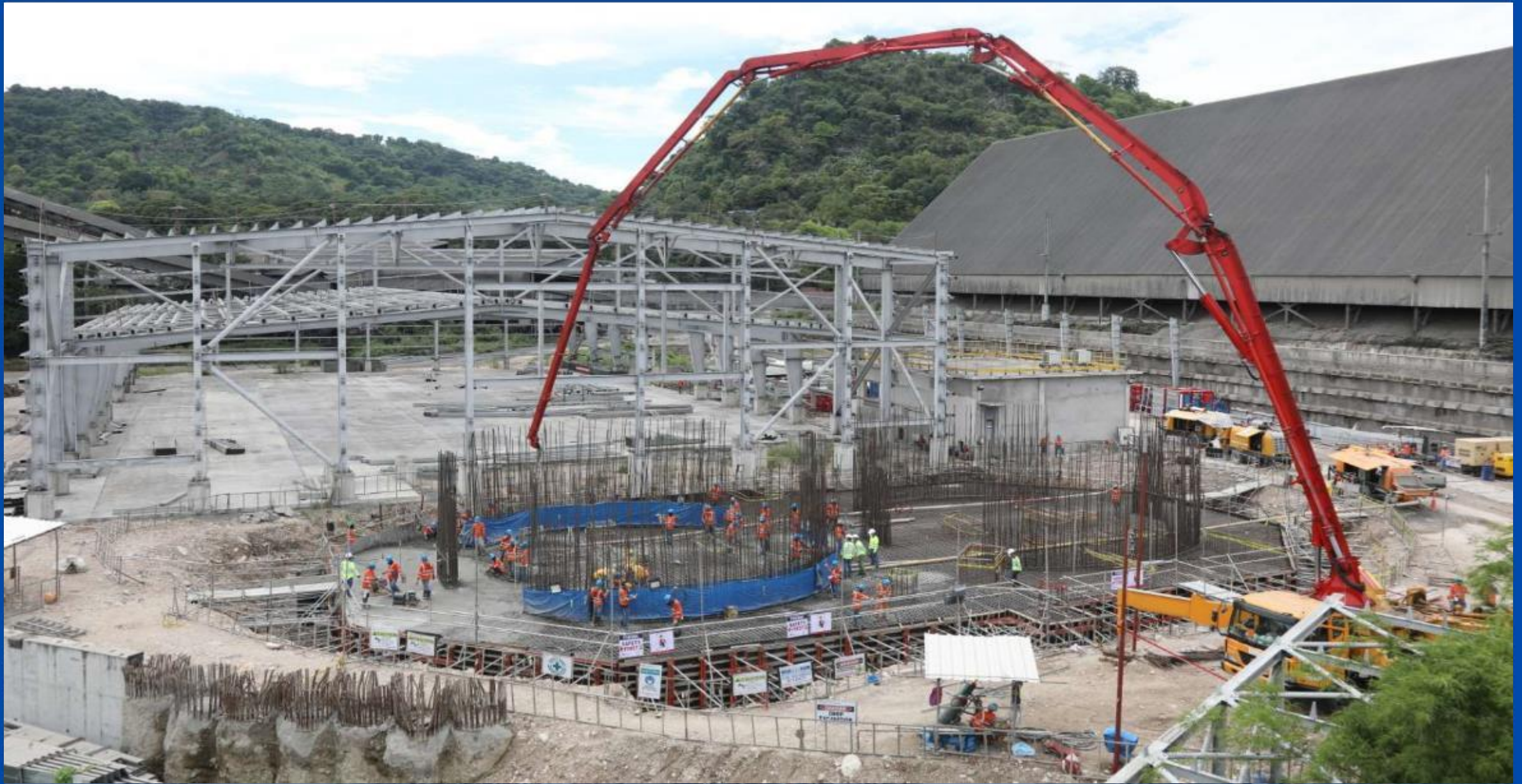
Concrete foundation pouring for cement silos in Solid Plant New Line project Built with Rizal Vertua® Classic High Strength cement
